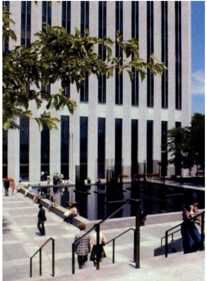
The plaza of the Standard Oil Building, Chicago, 1970s. Photographer unknown.
